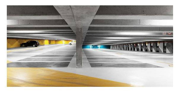
Example of lighting in a parking structure that does not extend below the structural beams. (Source: Aspect LED)
